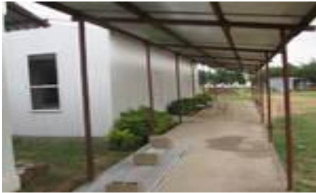
Covered walkways connect the wards and other buildings
